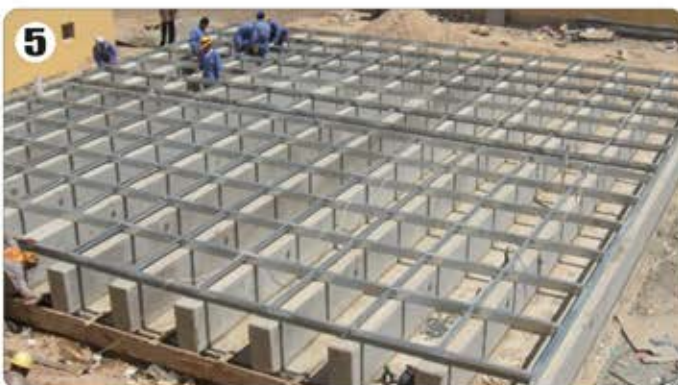
Concrete foundation for the erection of water tank
