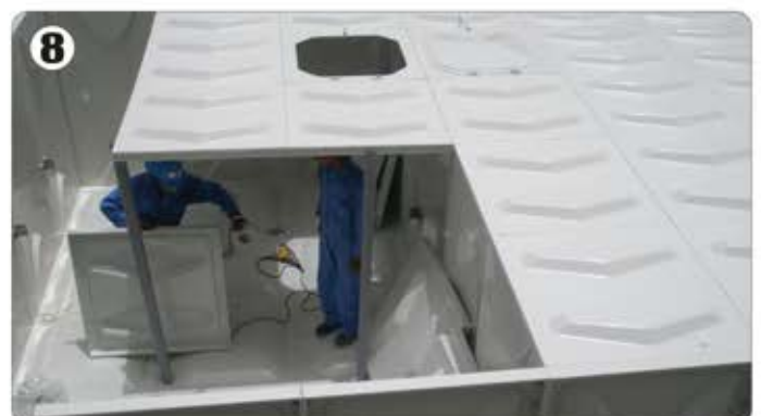
Assemble roof panel and manhole
