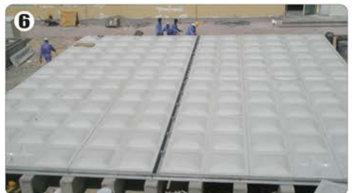
Assemble bottom panel
