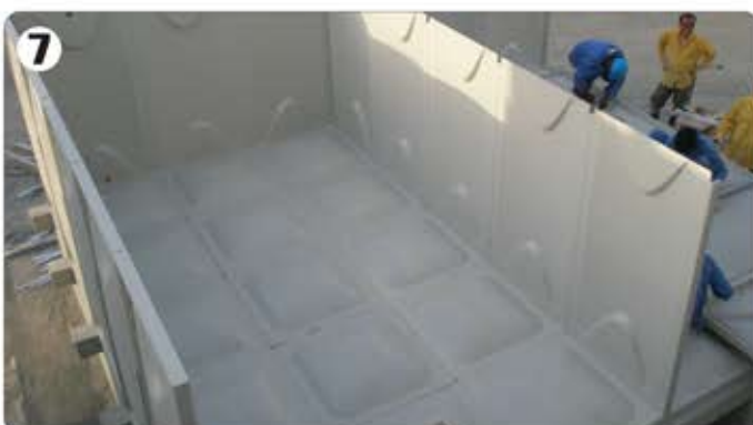
Erect wall and partition panel
